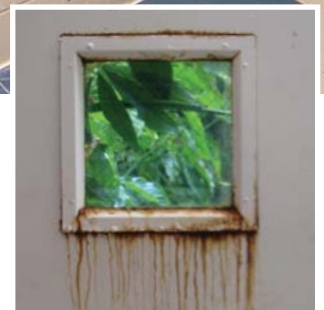
Hollow metal doors are not appropriate for corrosive environments.
