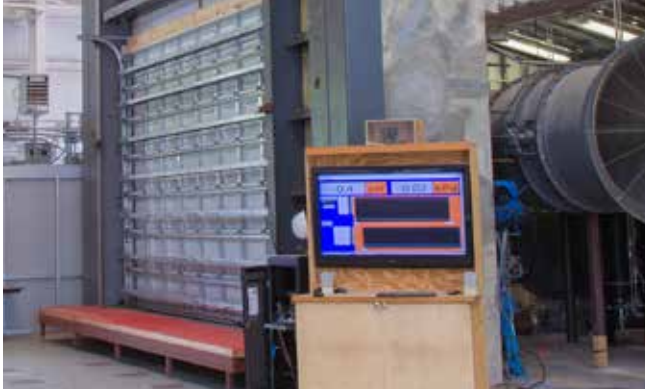
Sectional roll-up door installed prior to test.
