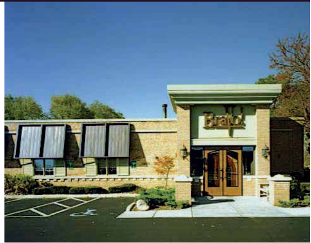
Eastern exposure puts the entrance to Bravo! in direct sunlight for nearly half of the day, which is no problem for the SL-19.
