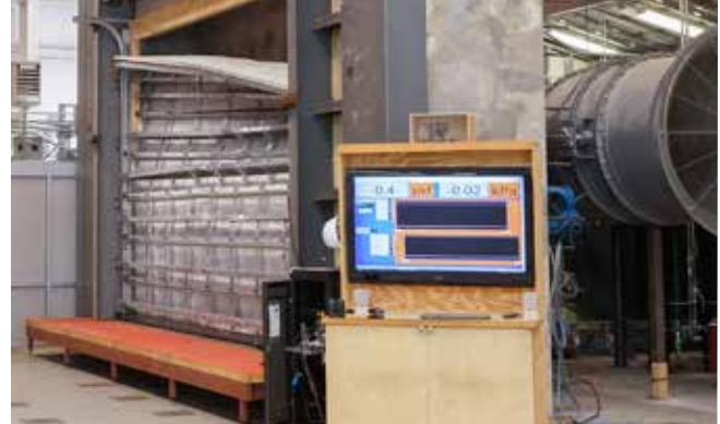
Damaged sectional roll-up door after test.
