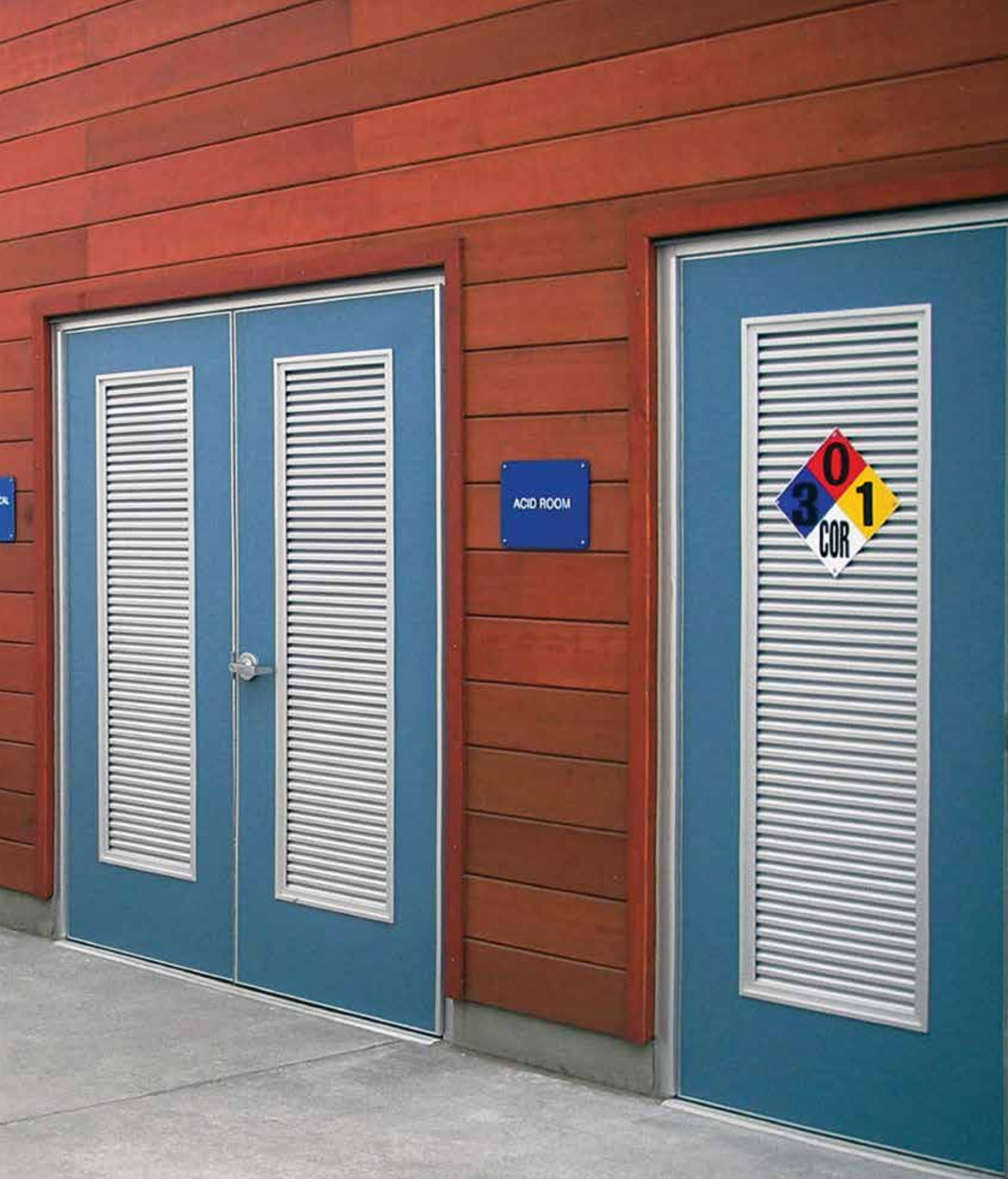
Fiberglass reinforced polyester (FRP)/aluminum hybrid doors (closed-cell foam injected) with aluminum louvers used for poolside chemical storage and mechanical rooms.
