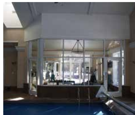
Below: Aluminum doors and aluminum-framed glass partitions at gym and pool area.
