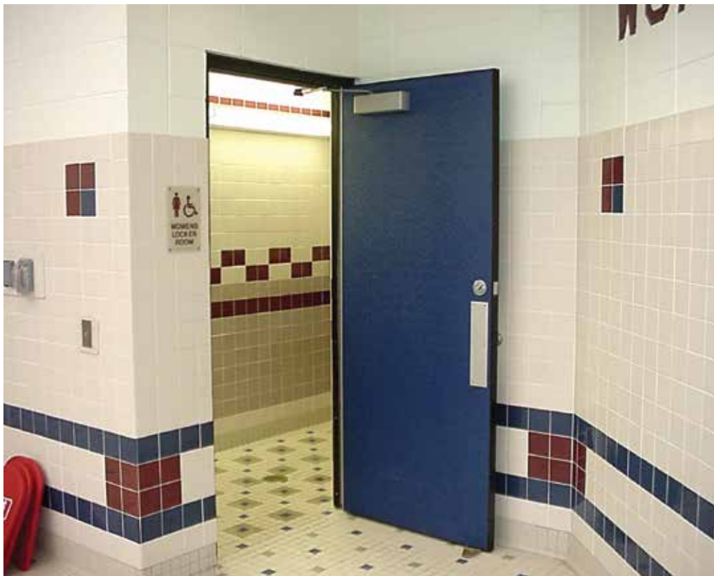
FRP/aluminum hybrid doors (closed-cell foam injected) used in showers in a pool locker room.
