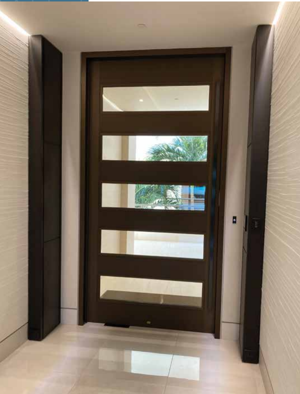
Left: An aluminum monumental door at a main floor entrance to a condominium in Hawaii.
