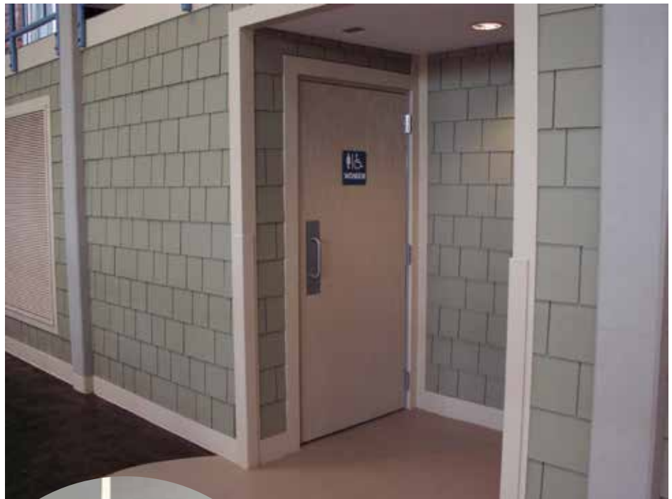
Wood grain FRP doors (closed-cell foam injected) at a motel.
