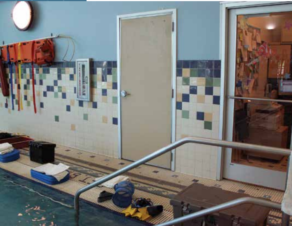
This FRP door to a fire-rated mechanical room at a pool features a stainless steel edge and a mineral core.
