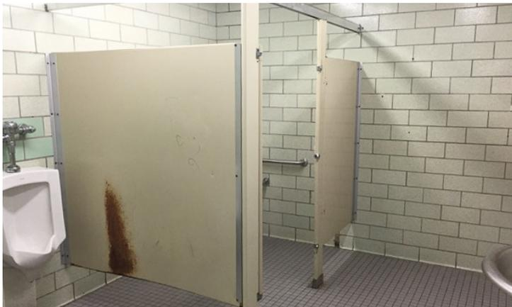
**BEFORE:** Exposure to liquids causes rust and creates sanitizing challenges. Metal panels have been bent and vandalized with permanent marker.
