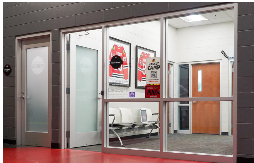
Interior Aluminum-Framed Glass Doors and Interior Aluminum Framing for a modern office area.
