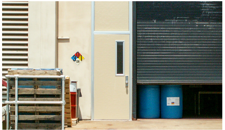
Hybrid FRP Door (SL-17) with Aluminum Tube Frame and FRP Architectural Panels.
