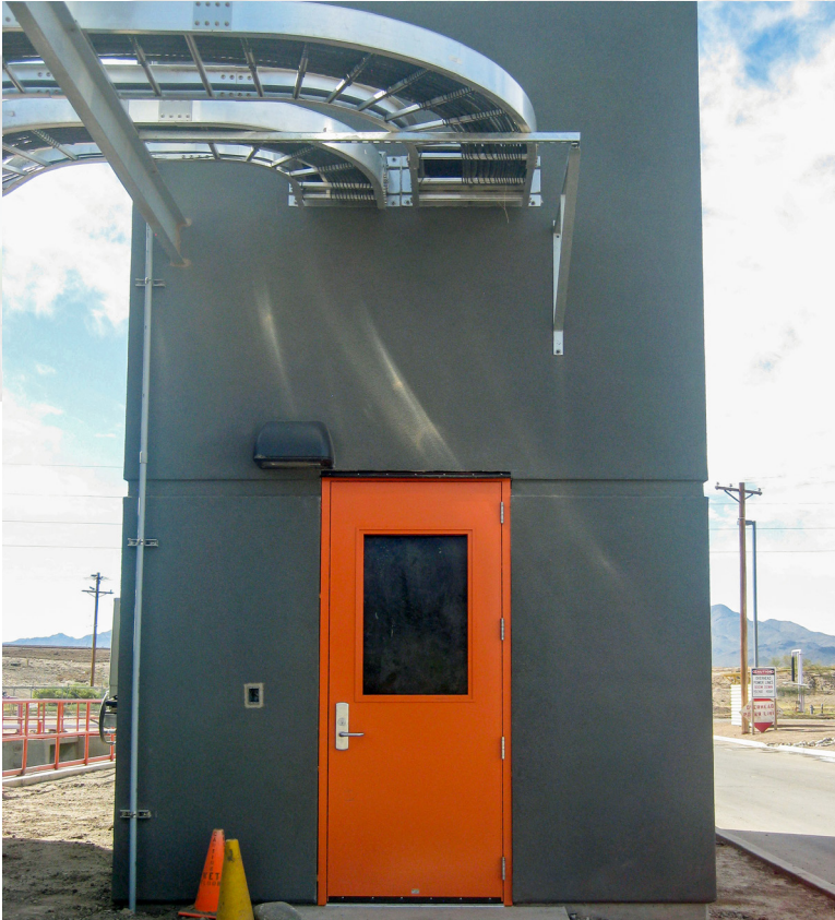
Aluminum Flush Door (SL-16) with painted finish - Ina Road Water Reclamation Facility in Tucson, AZ
