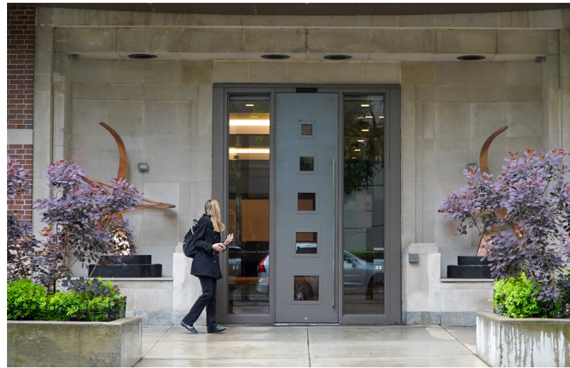
Chicago apartment building with extra-tall Aluminum Flush Door (SL-16) and graduated vision lite design.
