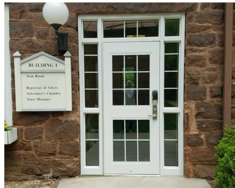
Monumental Aluminum Door (SL-15) on a municipal building.
